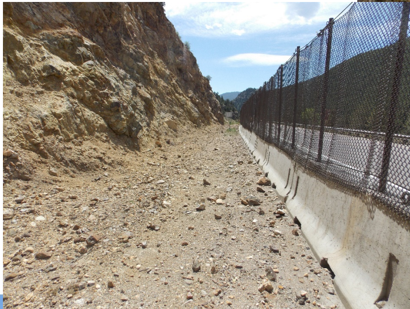
EXAMPLE: EXISTING ROCK CATCH DITCH JUST EAST OF DUMONT
